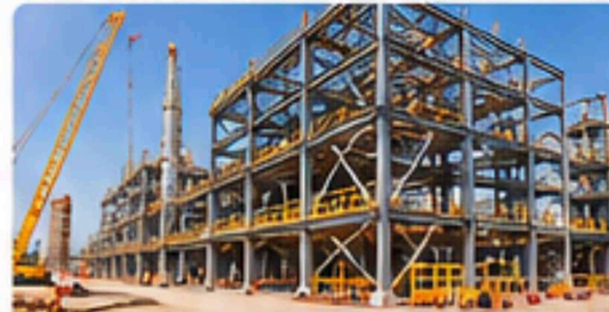
EPC and industrial construction
